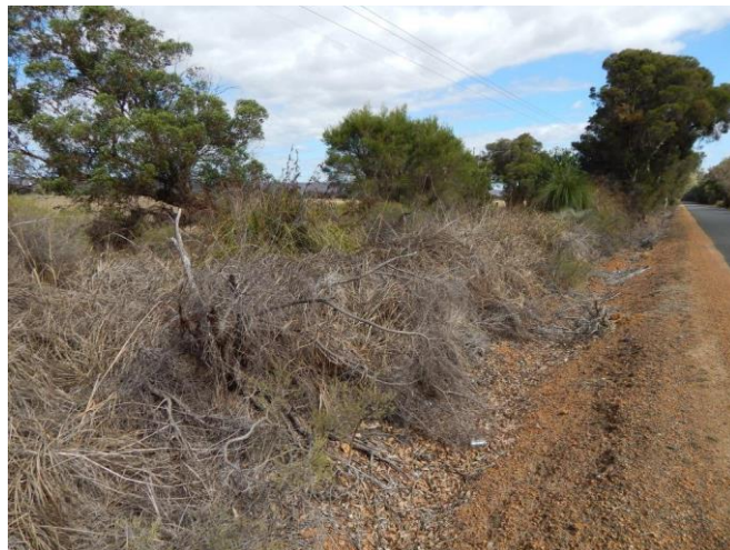
Figure 2. Poorly maintained road verge with heavy fuel load, Fawcett Rd Waroona
