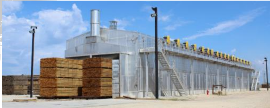
Source: American wood dryers
