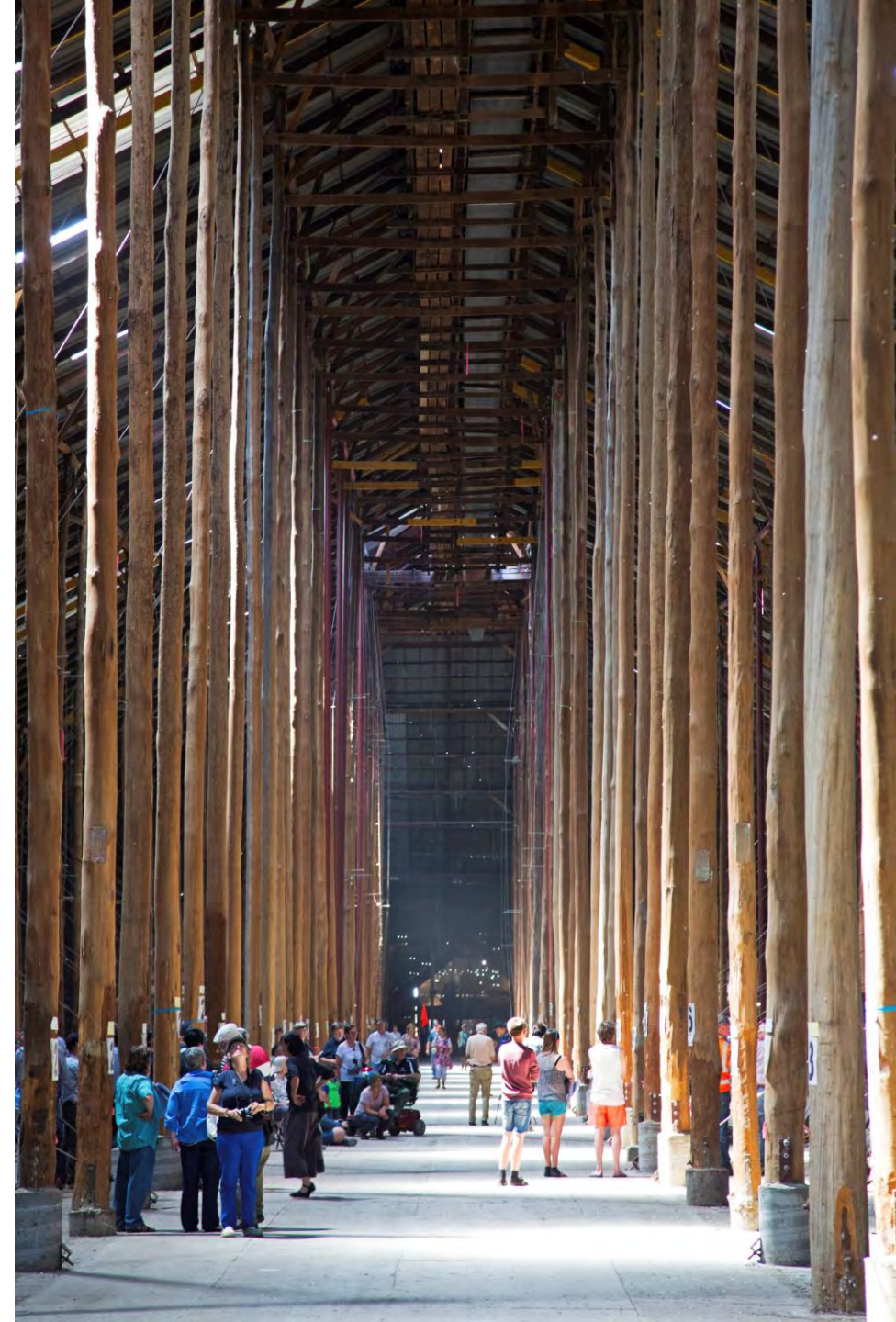
Right: Murtoa Stick Shed built in 1942 for grain storage using ash poles (photo M. Ryan)
